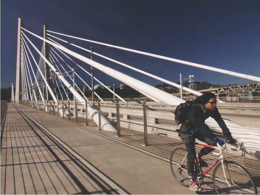
Portland's car-free Tilikum Crossing Bridge carries only trams, pedestrians and cyclists.
