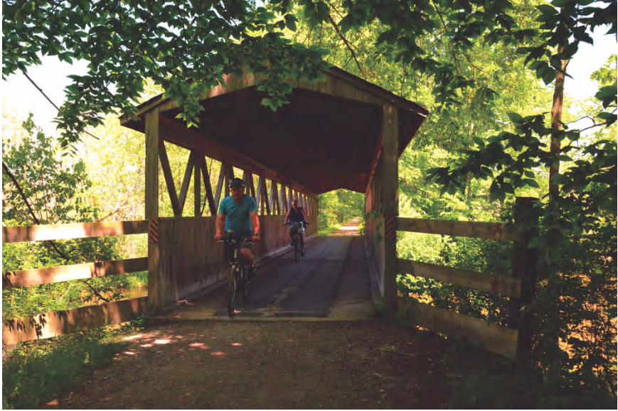
The Kal-Haven Trail crosses Black River on a covered bridge.
