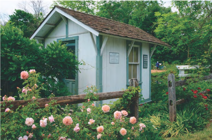
This bridge tender's station, built about 1830, is one of many canal-era structures still remaining on the D&R Trail.
