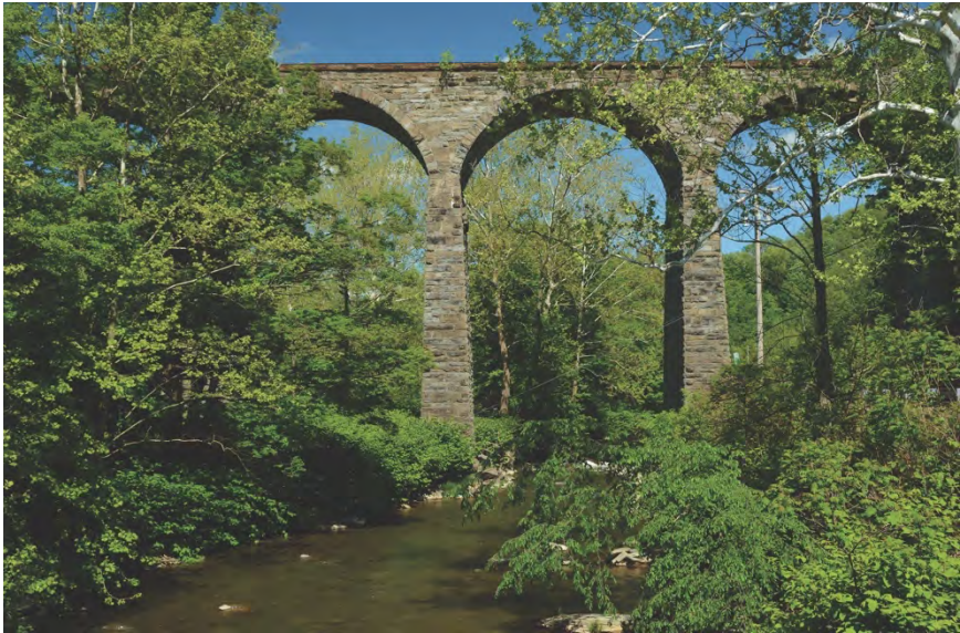
The Starrucca Viaduct, a thousand-foot-long stone arch bridge built in 1848, is still in use today.
