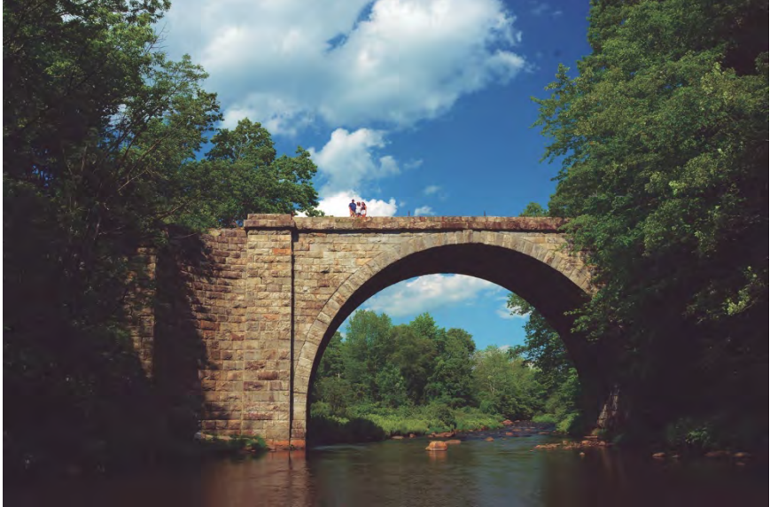
The 1847 Cheshire Railroad Stone Arch Bridge, now part of the Cheshire Rail Trail, is one of the best-preserved stone arch bridges of its era.
