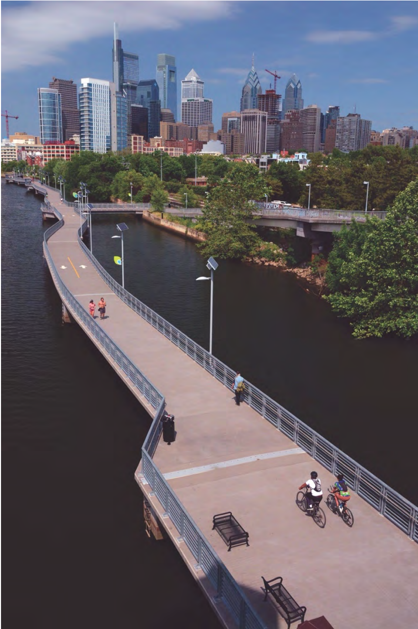
The Schuylkill Banks Boardwalk spans a segment of the river where the shore is too narrow to accommodate the trail.
